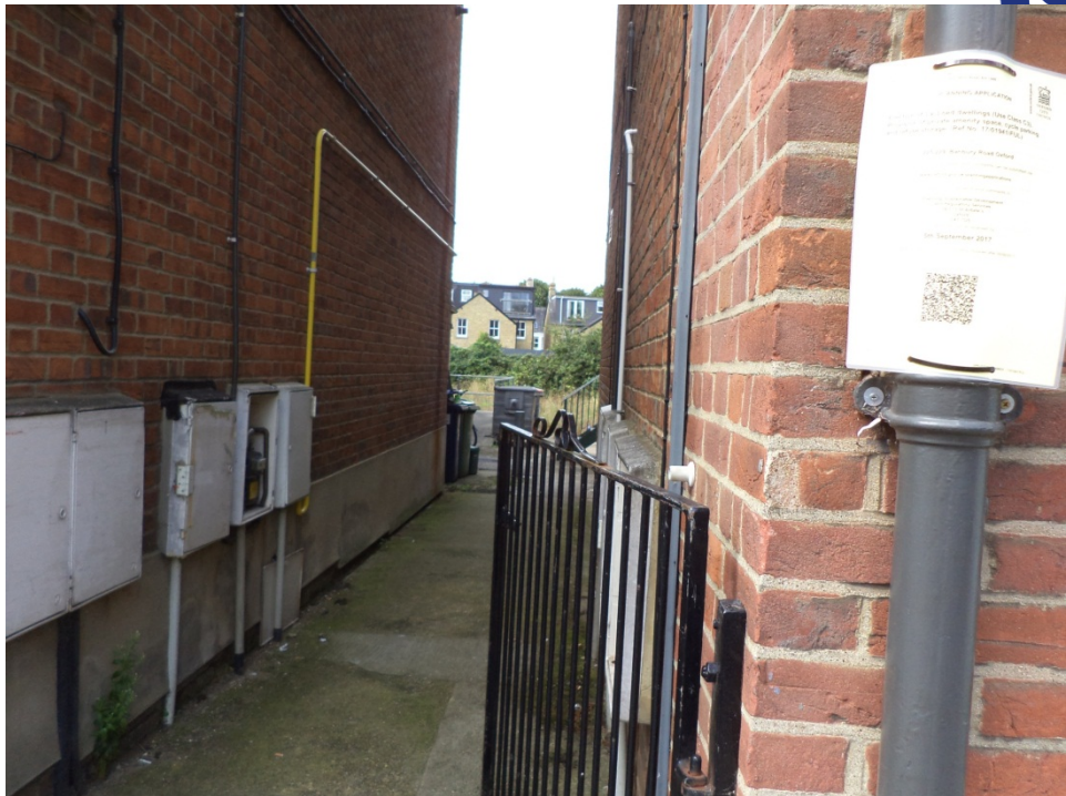
View of the existing access
